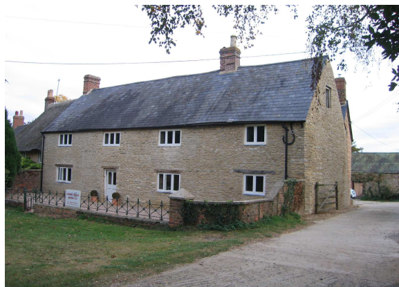
Montague Farm, Hethe (grade II), after restoration
