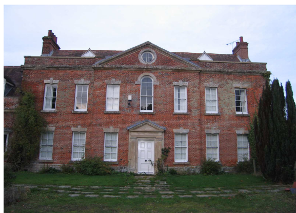
Finmere House (grade II), now undergoing a programme of repairs
