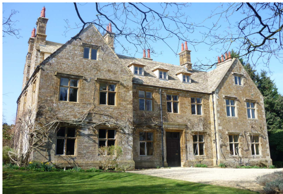
The Grange Adderbury, recently restored
