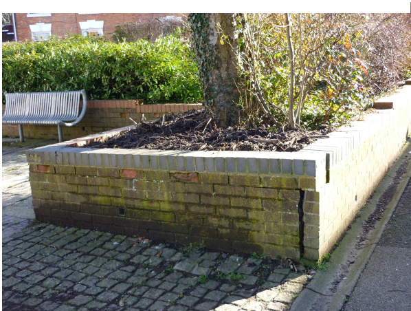
We have secured funding to work with Oxfordshire Highways and Banbury Town Council to undertake streetscape improvements in centre St and East St Grimsbury
