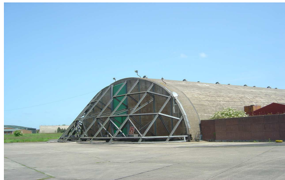
One of the 56 hardened aircraft shelters across the 505 hectare base at RAF Upper Heyford
