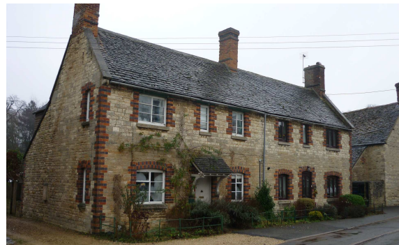
Springdale & Bishop's Cottage, undesignated heritage assets in Kirtlington; former Estate cottages where the window and door openings are framed in local red brick, with the burnt headers creating an attractive chequer board effect, that is highly locally distinctive.
