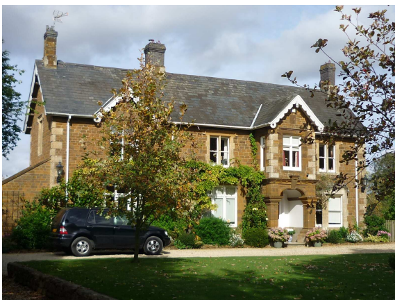
Holmby House, Sibford Ferris, nineteenth century gentleman's villa, an undesignated heritage asset
